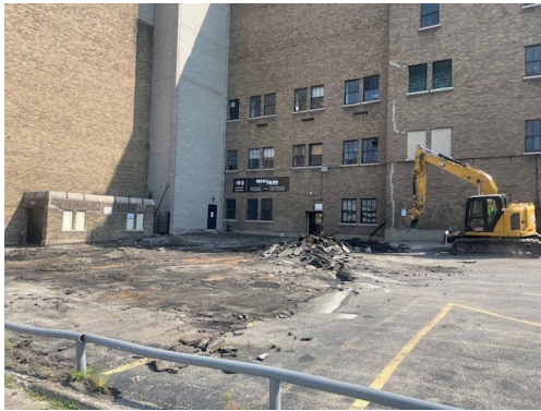
First Day of Demolition
